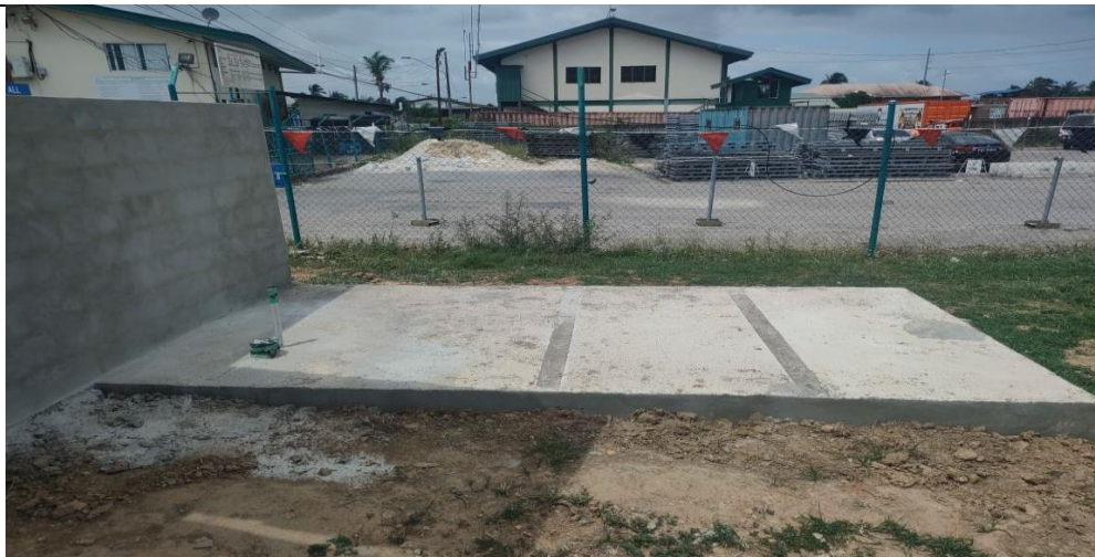
Figure 1 – Existing Plinth to facilitate housing of New Generator – Located near to the Main Entrance and Guard Booth area
